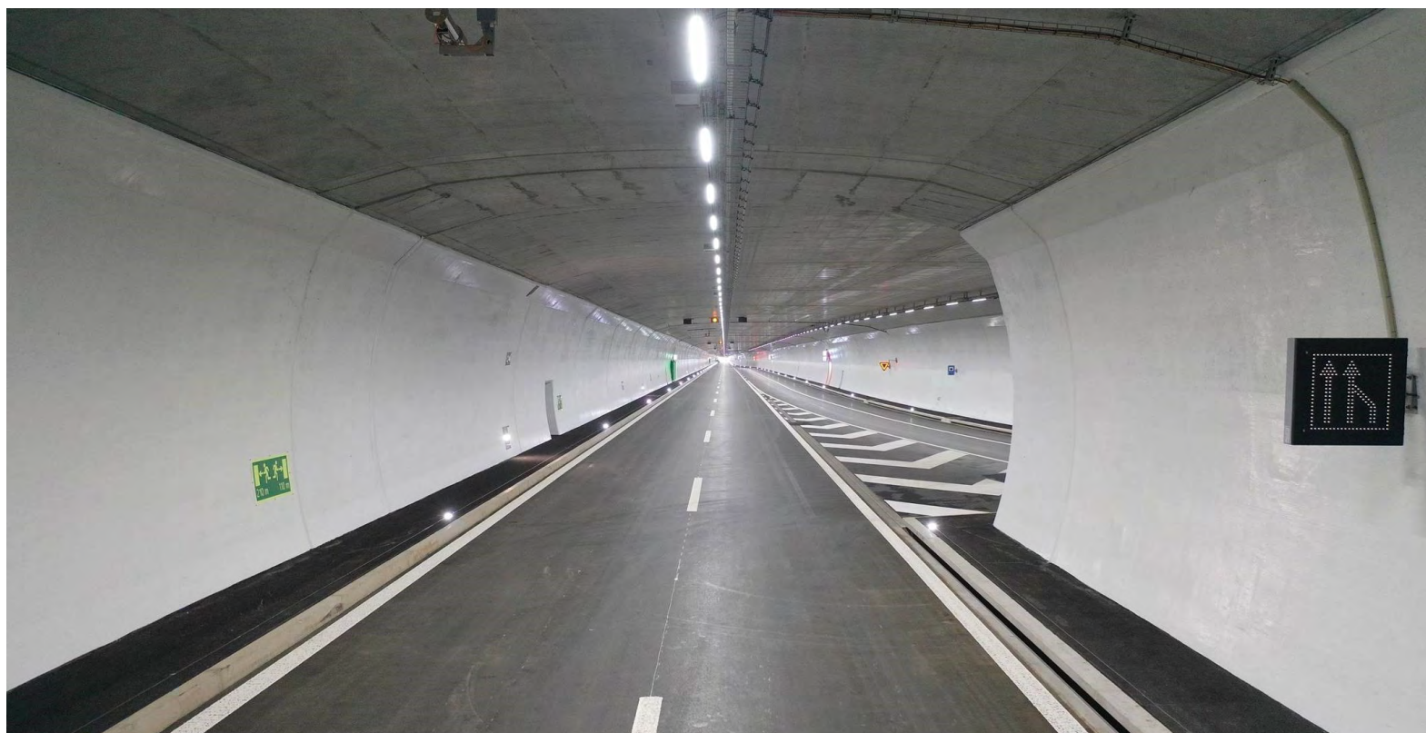
Tunnel Visp | Tunnel Visp
